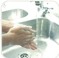
Sink Stainless Steel made
