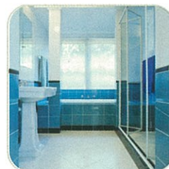
Bath Glaze tiles up to lintel level
